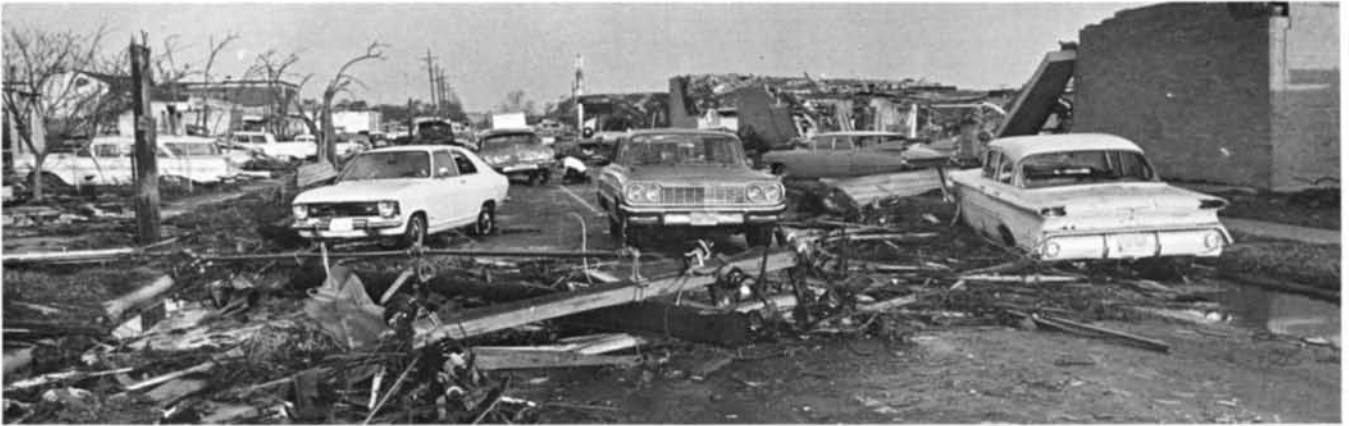
Fallen power poles block downtown streets.
